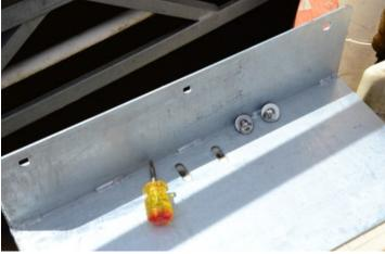
2. Mount the battery box bracket to the dock using the supplied ½" Phillips heads bolts and washers. Place the battery box on the bracket and mark the locations on the back of the box where the square holes are. Drill these locations. Mount the battery box to the bracket using the half inch carriage bolts, washers, & lock nuts.
