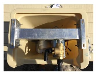
2. Using a 3/8" drill bit, drill through one wall nearest the bracket. TAKE CARE NOT TO DRILL THROUGH BOTH WALLS! This is to give clearance for a bolt, nut, and washer. Bolt the frame and bracket together using the supplied bolts, washers, and nuts. You may be required to unbolt the frame from the housing to complete this step.
